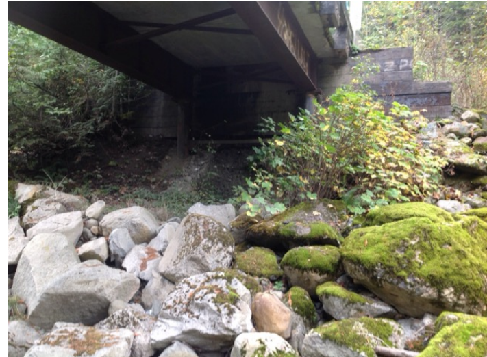
Right Bank Abutment when facing downstream
