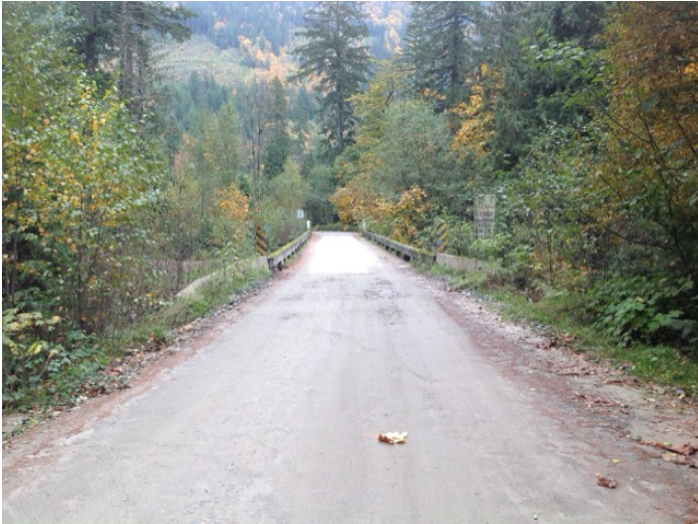
Approach from Right Bank when facing downstream
