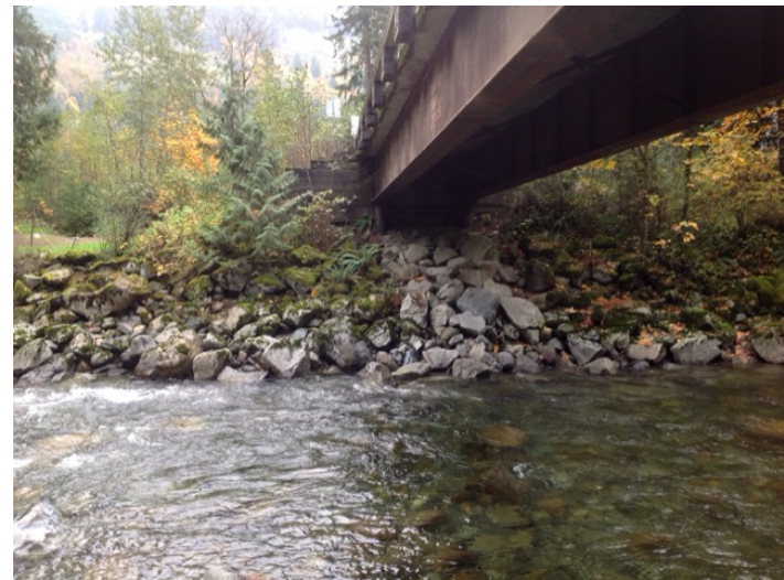
Left Bank Abutment when facing downstream
