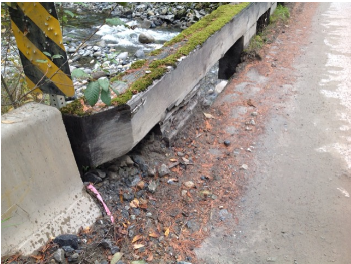
damaged riser
